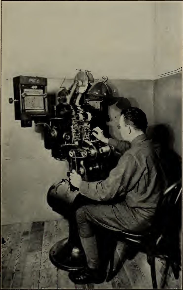
(Photograph by the Signal Corps School of Photography, U. S. A.)
